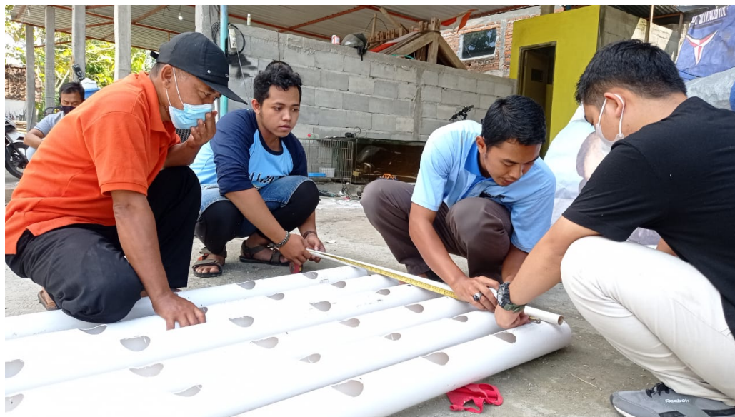
Gambar 2. Proses Pengukuran Lubang Pipa PVC
